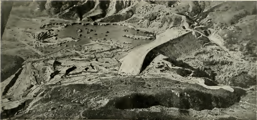
Dam is typical rolled-earth-fill structure with impervious upstream portion and pervious downstream section.
